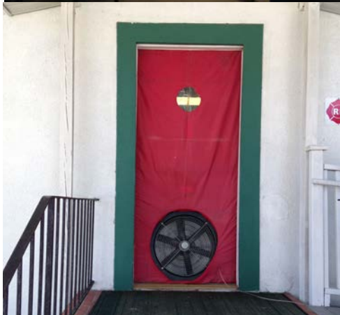
Energy Efficiency workshop at Flowers Temple, taught by Kris Stenger. Below, Duct Test prior to retrofit at Flowers Temple Annex. Photos: Deborah Green
